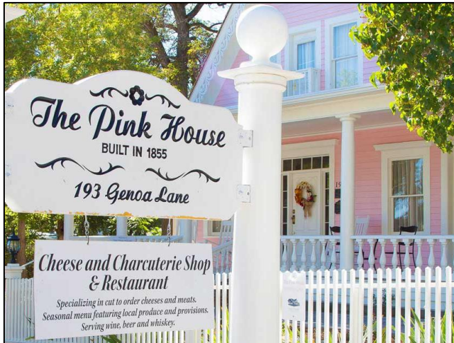
The Pink House in Genoa utilized rehabilitation tax credits
