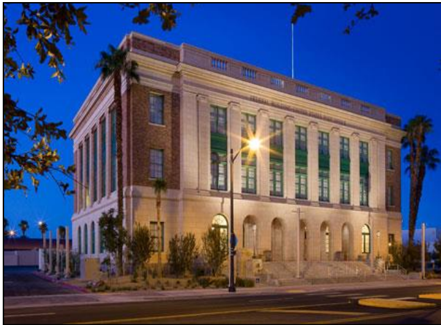
1930 Las Vegas Post Office and Courthouse Tax credits earned during conversion to Mob Museum
